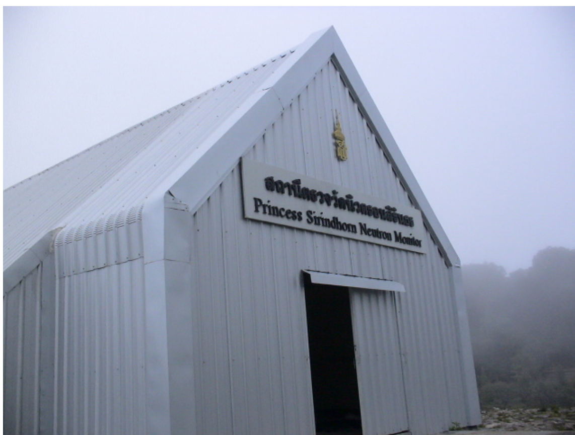
Figure 8: The Princess Sirindhorn Neutron Monitor after additional construction in April, 2010.
