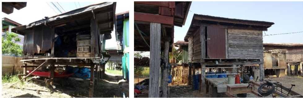
Figure 5.32: Small huts are special buildings found in Ban Rangnok which are used as storage spaces for keeping domestic stuff (ground floors) from flooding
