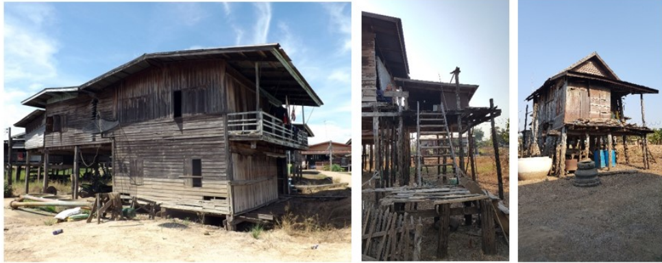
Figure 5.31: Wooden walls were built in horizontal rather vertical aligned pattern which can be repaired and replaced easier after flooding (left). A rope used for carrying things from ground to upper elevated floor during flooding (middle). Stilt structure was applied to other types of buildings, a small rice granary is a case in point (Right)
