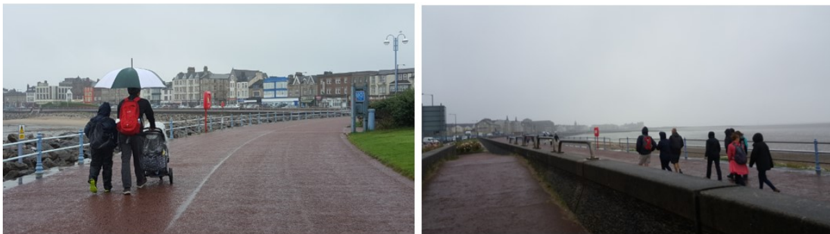
Figure 6.13: Existing Seawalls along Morecambe Bay in Lancashire, UK
