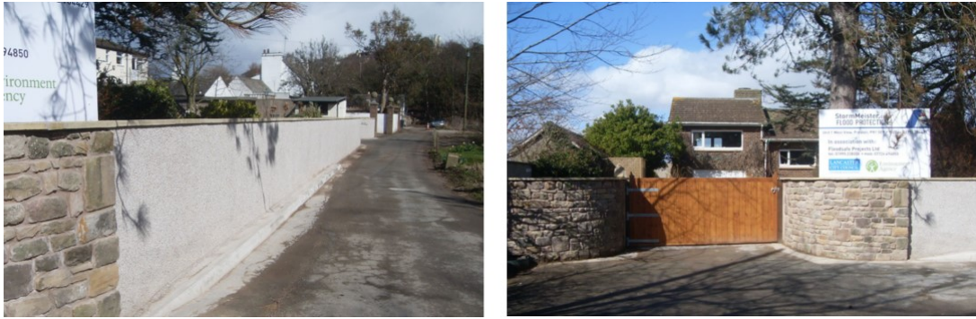
Figure 6.6: Floodwall protection from tidal surges by Lancaster City Council http://www.floodsafeprojects.co.uk/portfolio_page/flood_walls_council_lancashire/
