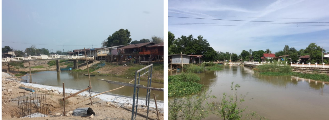
Figure 5.16: Some parts of riverbank were replaced by concrete embankment
