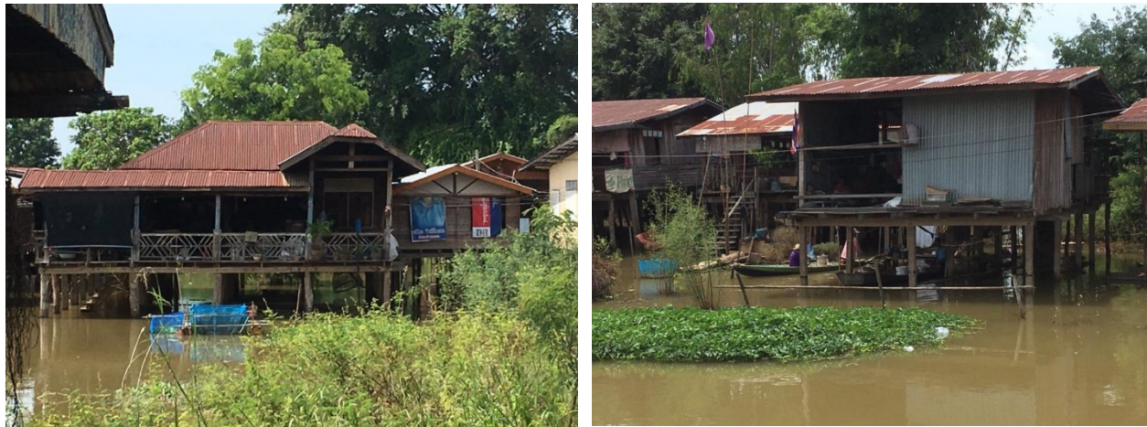
Figure 5.17: Traditional Stilt Houses. The only one stilt house with gable hip roofs remained by the Yom River in Ban Kong (Left). Most of stilt house with gable roofs are common housing characteristics in tropical climate (Right) (Photo by Pittungnapoo W., 2017)
