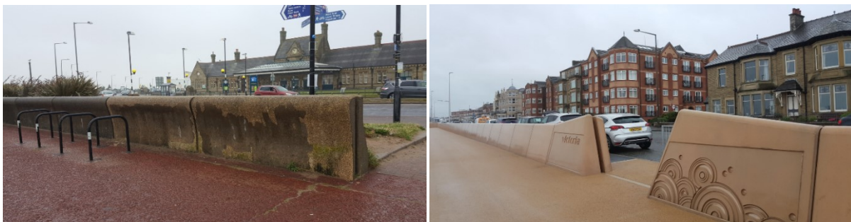
Figure 6.14: Existing Seawalls (Left) and New Replacement of Sea Wave Reflection (Right) in Morecambe, Lancashire, UK (Photos by Pittungnapoo, W., July 2017)
