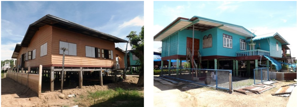
Figure 5.29: Walls are not common building elements found in Ban Rangnok One side of wall built to protect flood (Left) Clear fences built to define space underneath the stilt house which try to avoid visual block (Right)
