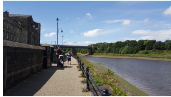
Figure 6.5: Green embankment in Rotterdam (Left) A combination between flood walls and green embankment as a mixed measure of flood mitigation by the River Lune, Lancaster: UK (Right) Photos by Pittungnapoo, W., July/ 2017)
