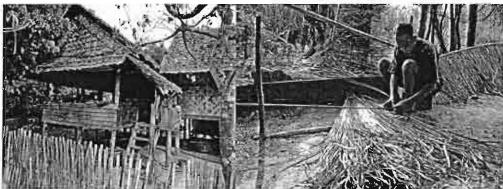
Fig 4.16 Thatch Roofs, weaving and binding method.
