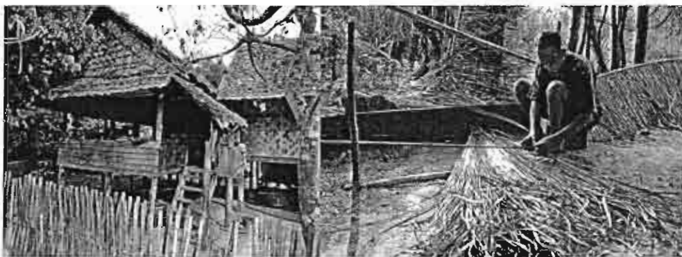
Fig 4.16 Thatch Roofs, weaving and binding method.
