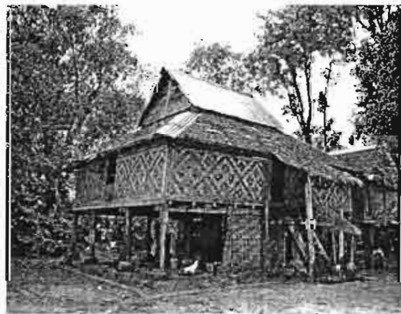
Fig 4.3 Thai Vernacular House with mat-like enclosure
