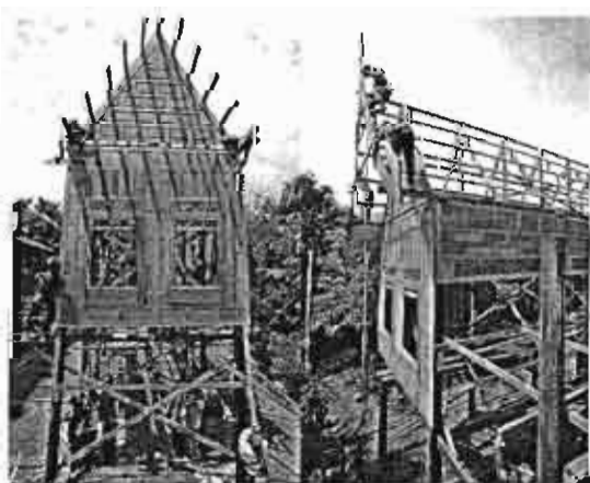
Fig 4.10 Wall panels put into place
