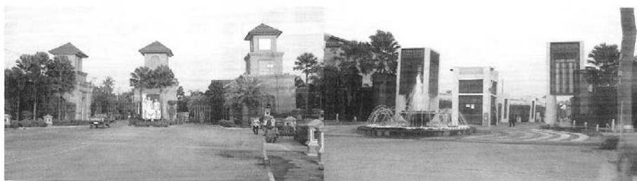
Fig. 8. Photographs showing entrances of two gated communities Source: Karnchanaporn and Kasemsook
