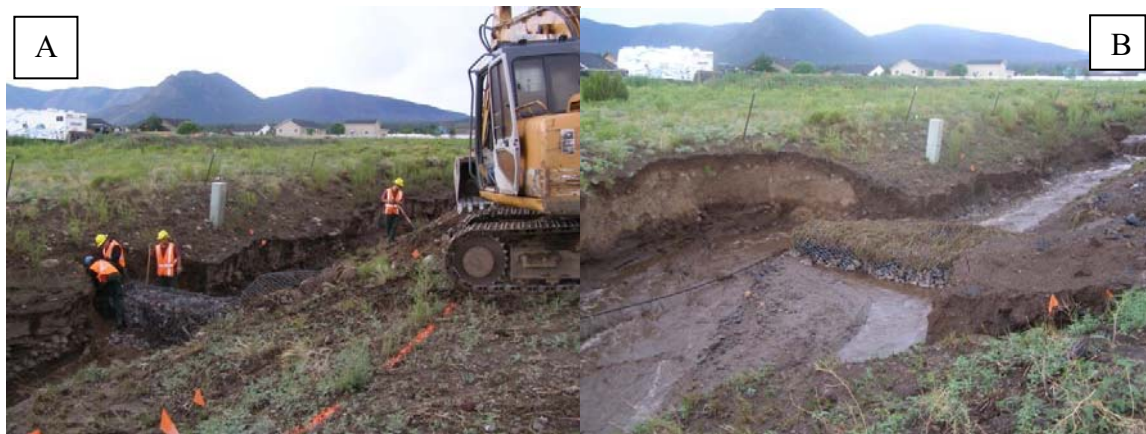
Figure 3. Gabion construction along Campbell Avenue prior to the July 30, 2010, storm (A); and results during the storm event showing gabion failure and channel widening (B).
