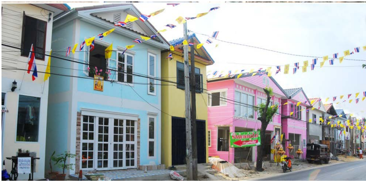
Figure 3 the new-built housing in Chumchon Bang ra-mard. The nearby space around the house is reduced.
