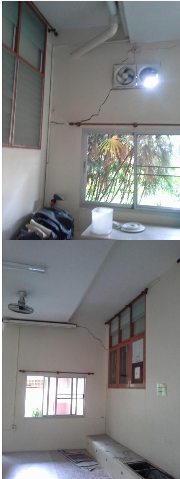
รูปที่ 1. Observed cracks on infill wall if the ground shaking was larger this wall would collapse inside the buildings.
