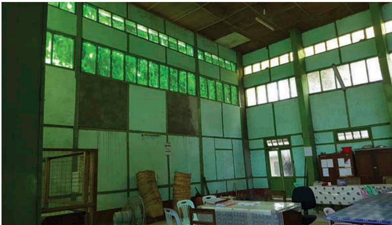
Figure 9. Timber frame with brick noggin is widely observed in Bagan and Chauk without any structural damage; however, nonstructural failures such as out-of-plane failure of brick wall and ceiling were observed in Chauk.
