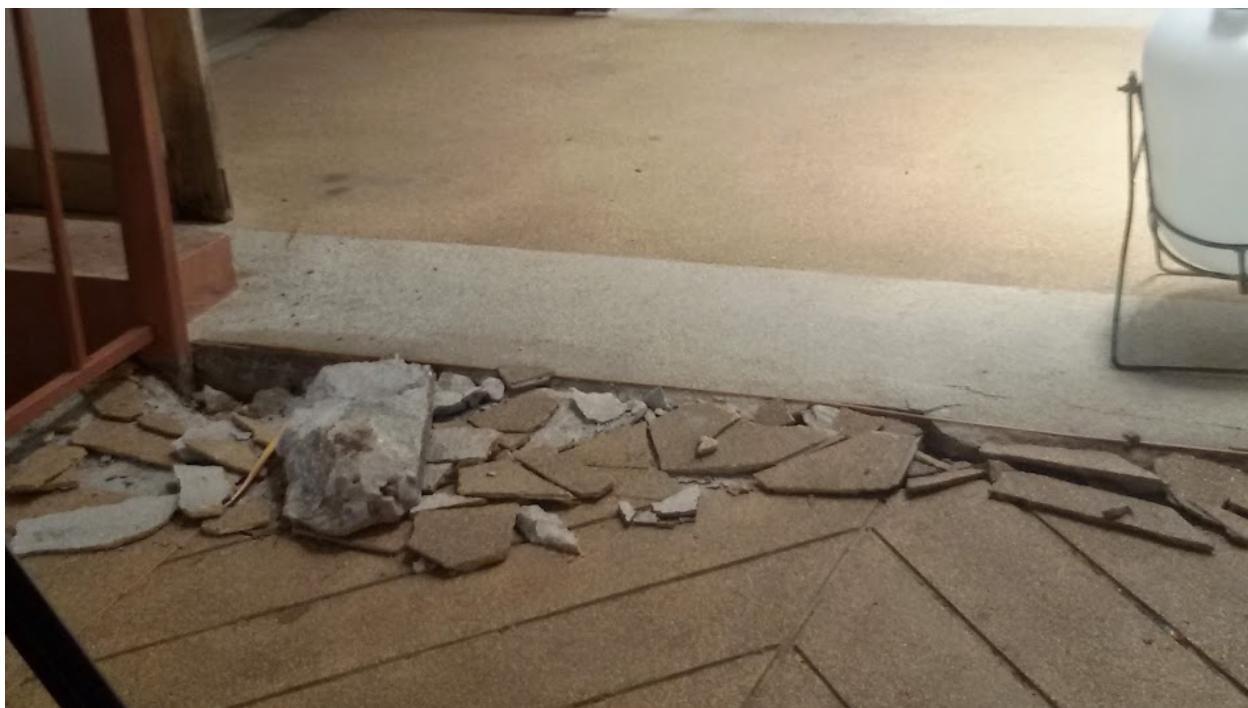
รูปที่ 2. Observed cracks between two adjacent buildings since there is very minimum distance between these two structures.
