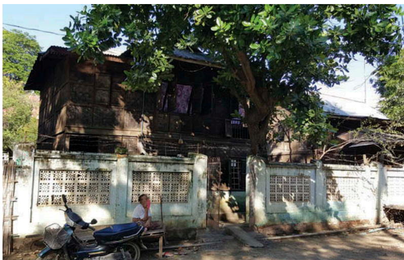
Figure 10. Wooden frame with mat infills is widely used in Chauk and Bagan without any structural and nonstructural damage since it is light and more flexible. Most of these kinds of structures are usually one- or two-story buildings.
