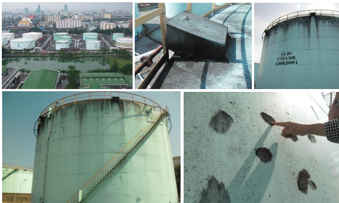
Figure 1 | Aspergillus niger strain ES4 growing on the roof and outside upper wall of an ethanol tank of a petroleum company.
