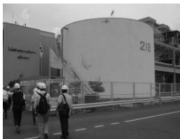
EGAT's Power Plant
