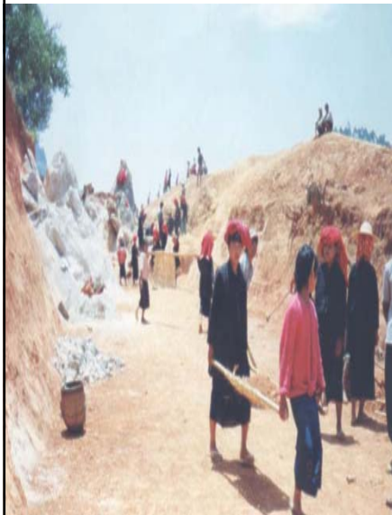
Rail way construction
