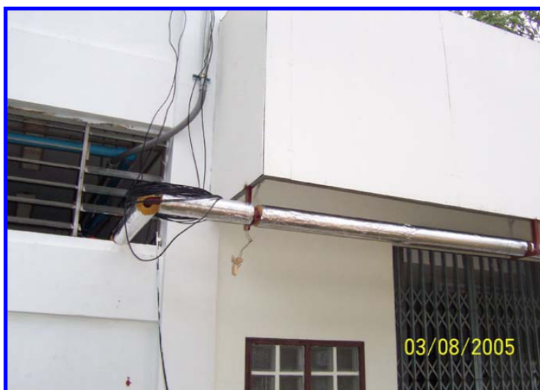
Figure 3.7: Routing of the steam pipe from inside the Department of Chemical Engineering.
