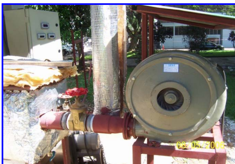
Figure 3.8: High pressure blower for injection air passed the superheater into the drying kiln.
