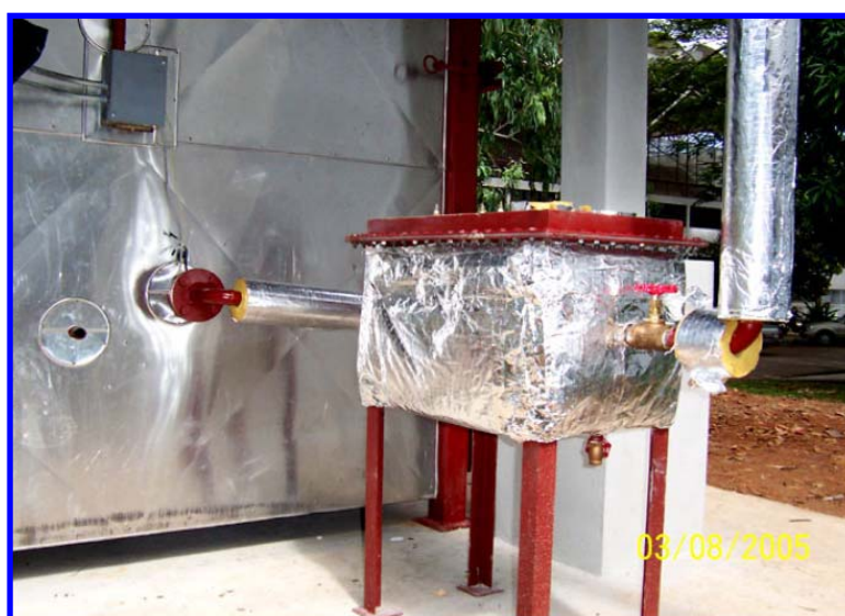
Figure 3.4: A super heater located next to the piping entrance into the chamber.
