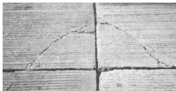
Corner Crack
