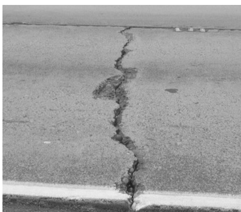
Transverse Crack
