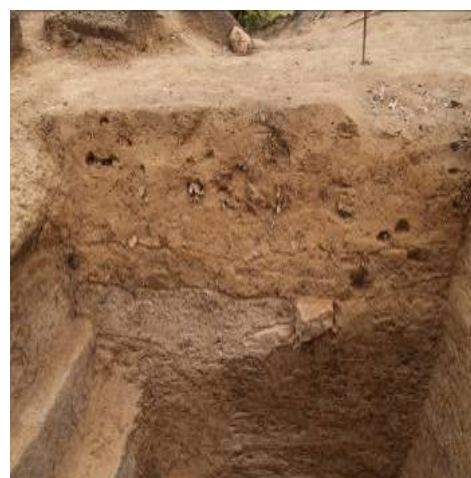
Fig. 6-25 Compacted soil layers at bridge's head
