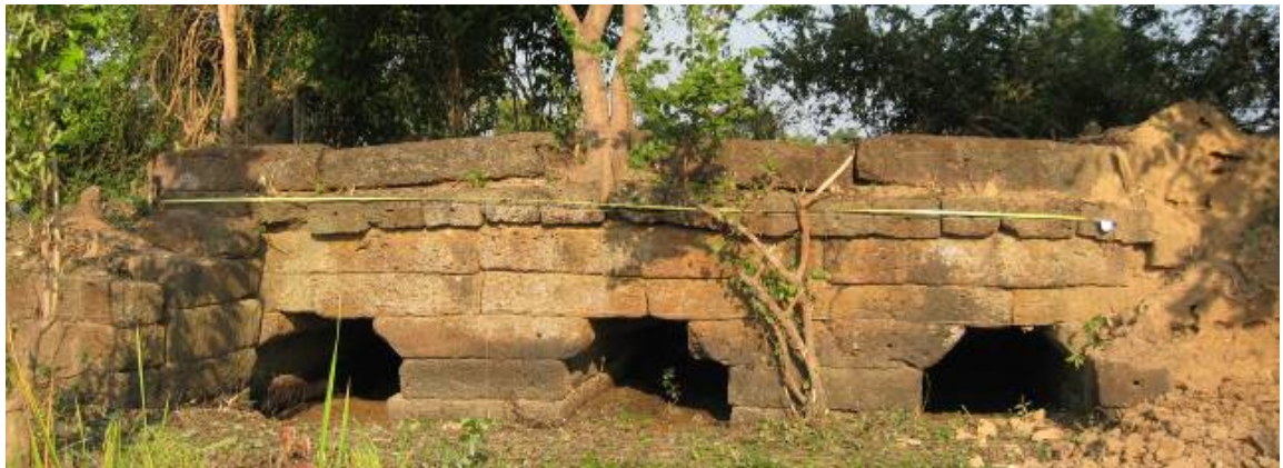
Fig. 6-21 West facade elevation view
