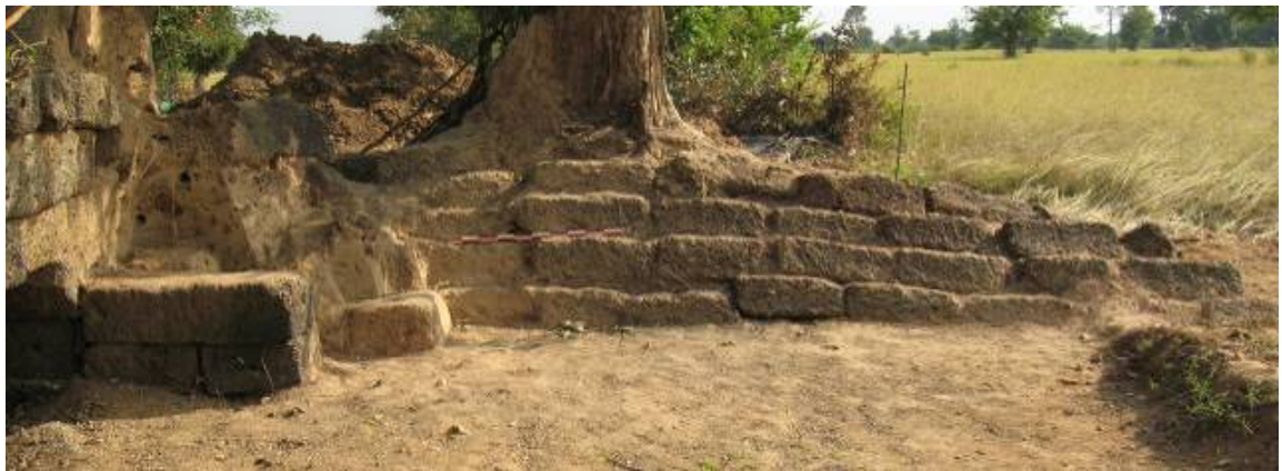
Fig. 6-20 View of retaining wall and wing wall
