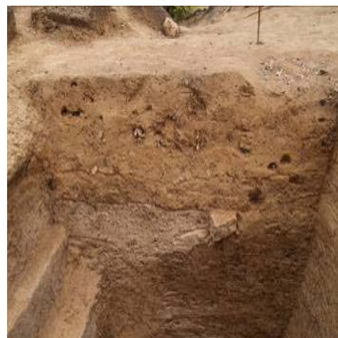
Fig. 6-25 Compacted soil layers at bridge's head
