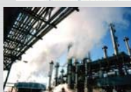
Chemical Plant explosion in Seveso, Italy
