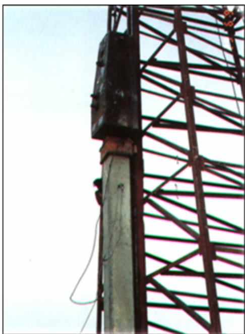
Initial Driving Test
