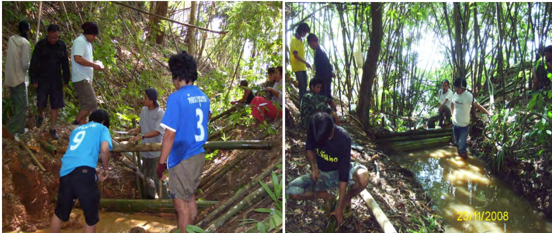
Figure 2.12 Construction of Check Dams for Water Conservation ( source : GEF/UNDP report , 2010)
