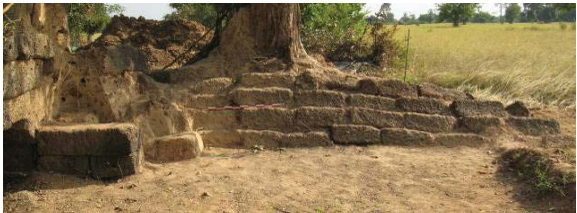
Fig. 6-20 View of retaining wall and wing wall
