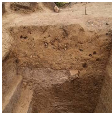
Fig. 6-25 Compacted soil layers at bridge's head
