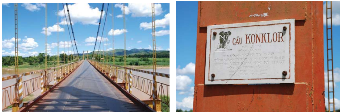
Fig. 5.19 Kon Klor bridge built in 1994
