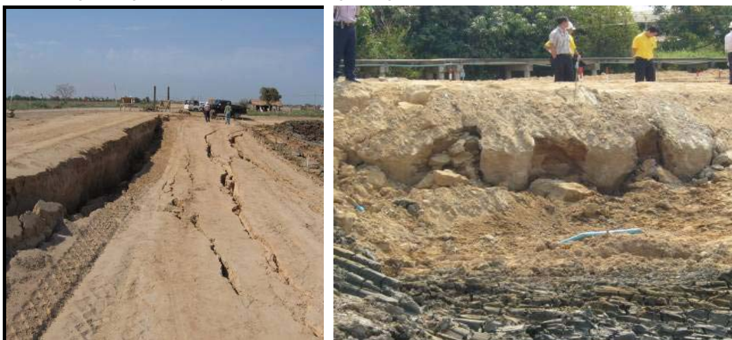
a) Stability failure
