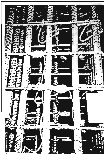
Fig. 6 Column reinforcing cage with hook clips in place.
